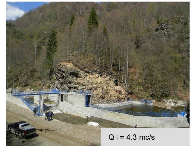
Water intake Sadu A on Riverl Sadu, county Sibiu
