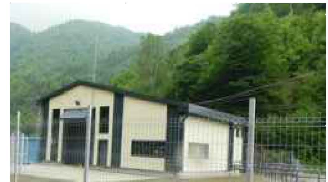
HPP Sadu A - Exterior View
